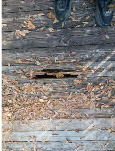
Pic 1 shows current condition of decking
